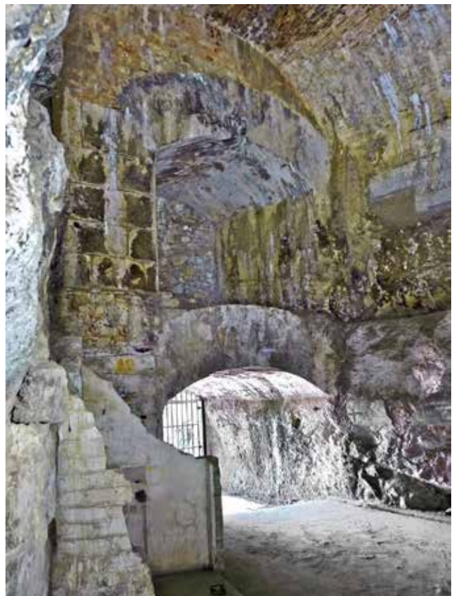
The two-storey casemate of Upper Orillon Battery, exploiting a natural fault
